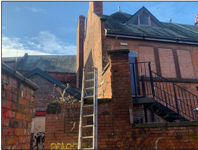
Localised Area to Proposed Mechanical Plant
