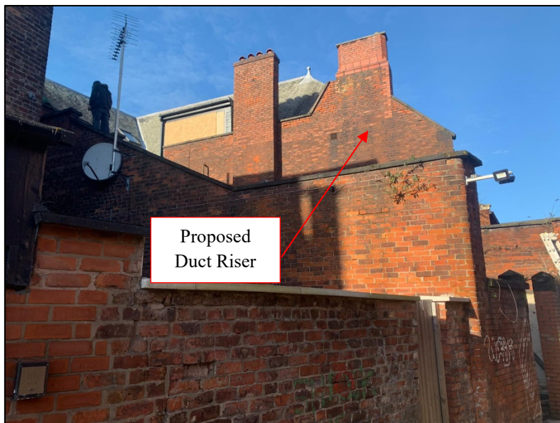
Localised Area to Proposed Mechanical Plant
