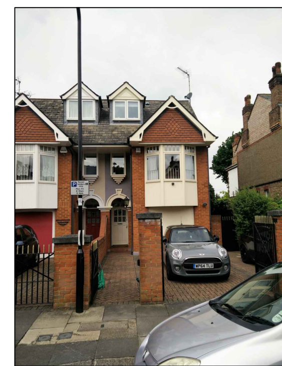
EXISTING FRONT PHOTOS
