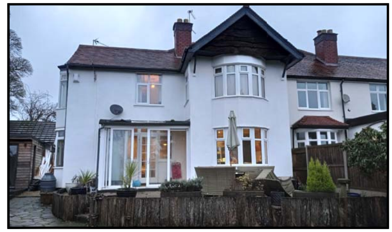
REAR ELEVATION PHOTOGRAPH
