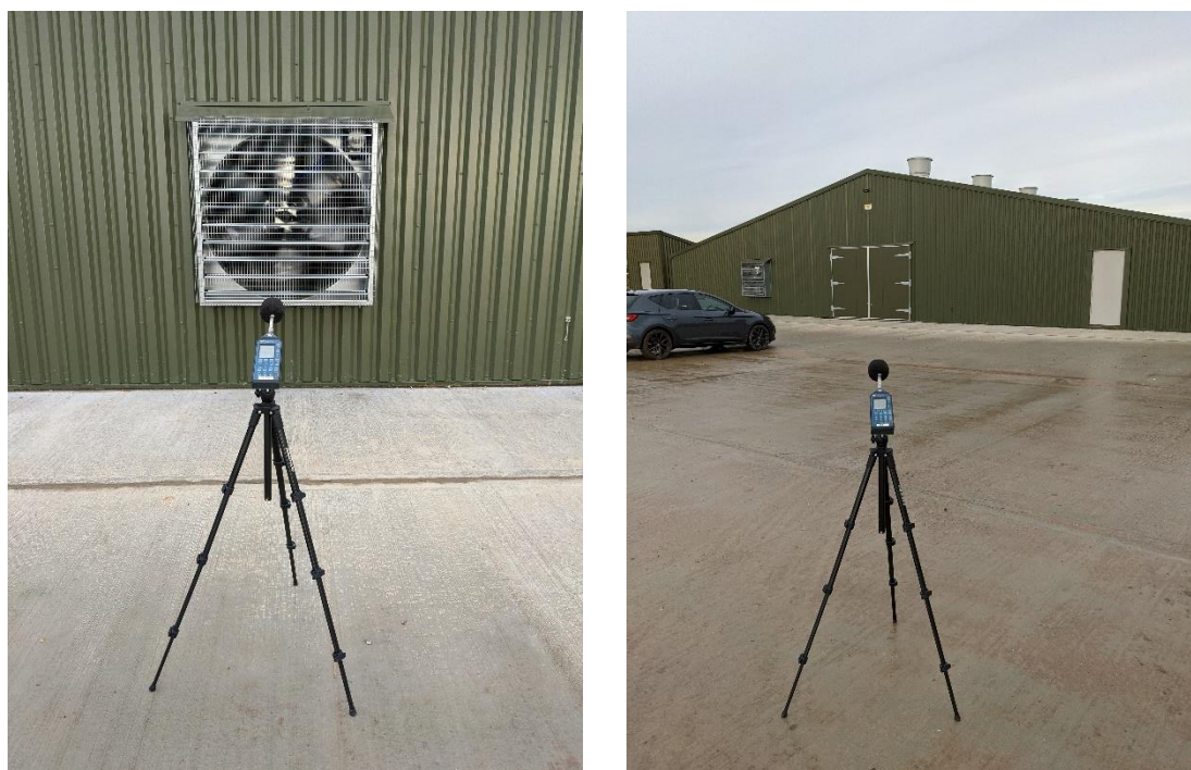
Figure 3 – Photographs of gable (left) and chimney (right) fan measurement positions
