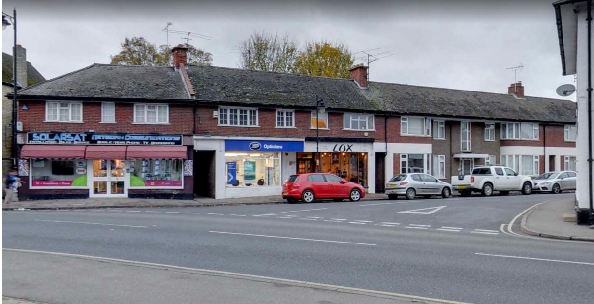
View of Shop Frontage (LOX) as existing from High Street
