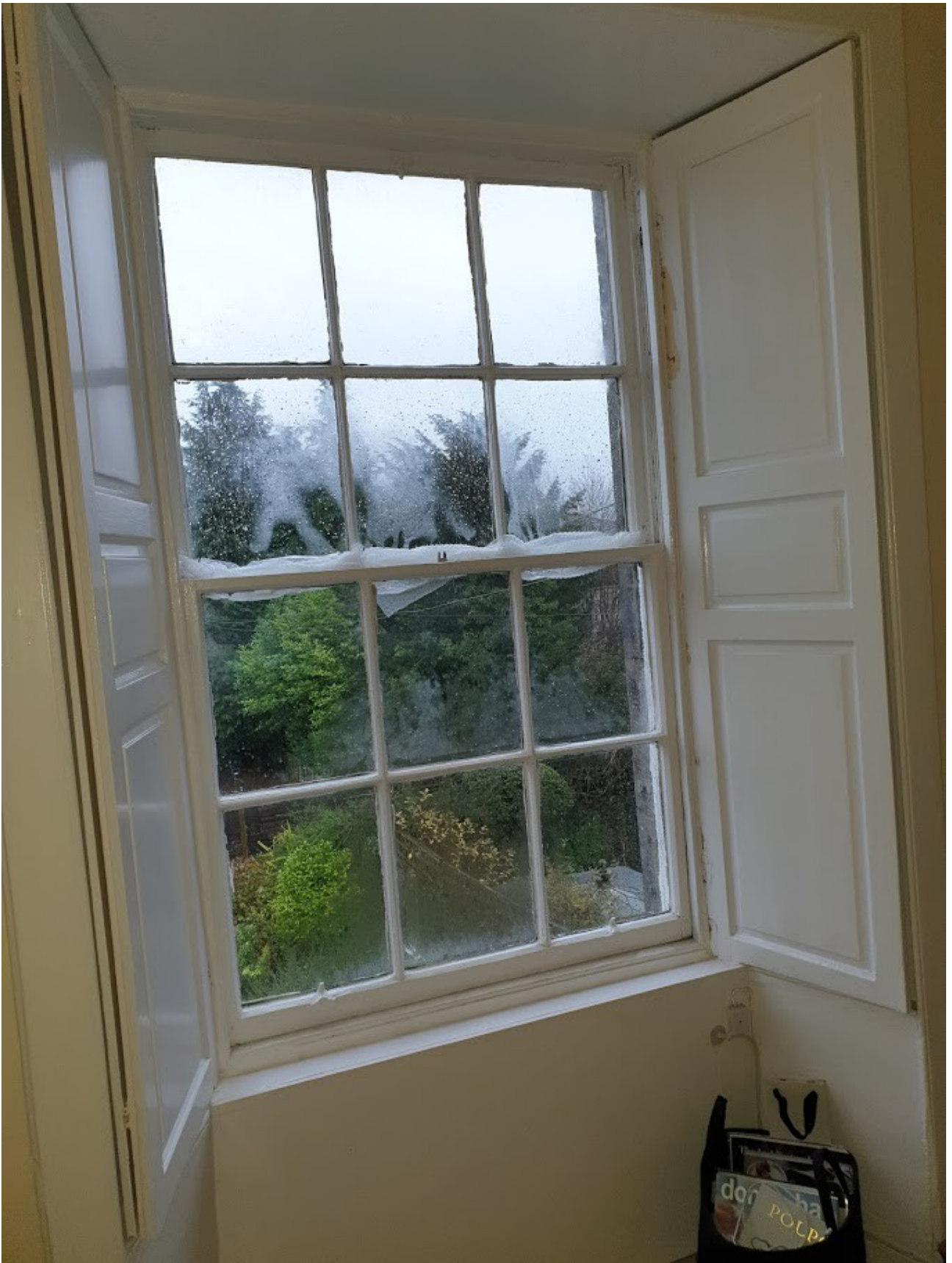
EXISTING SINGLE GLAZED WINDOW IN DINING AREA
