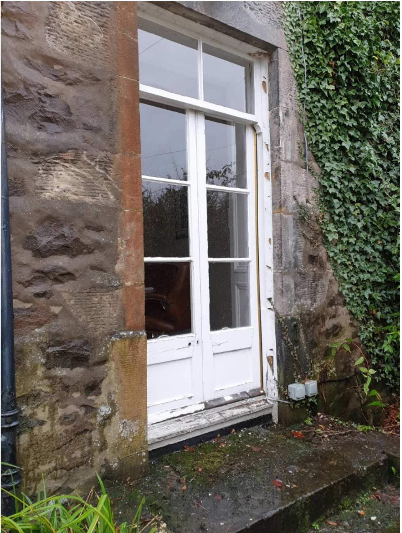
EXISTING EXTERNAL PATIO DOORS OF LOWER PROPERTY
