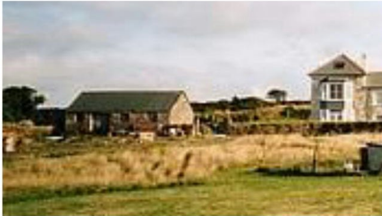
Fig 1; Northern aspect and converted workshop
