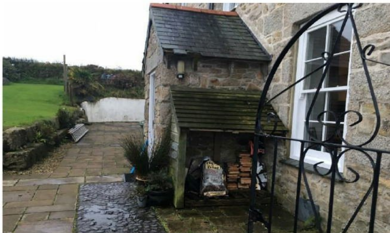
Fig 2; Existing entrance to the Count House
