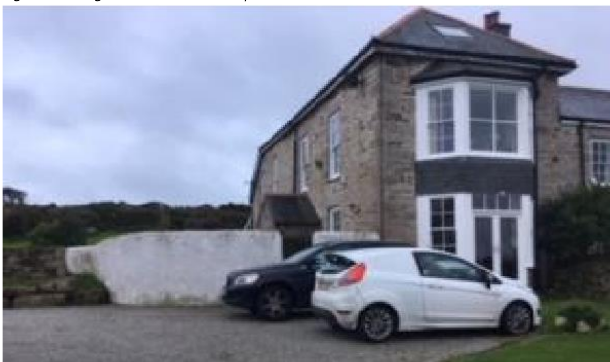
Fig 14 Existing rendered garden wall adjoining the north elevation.
