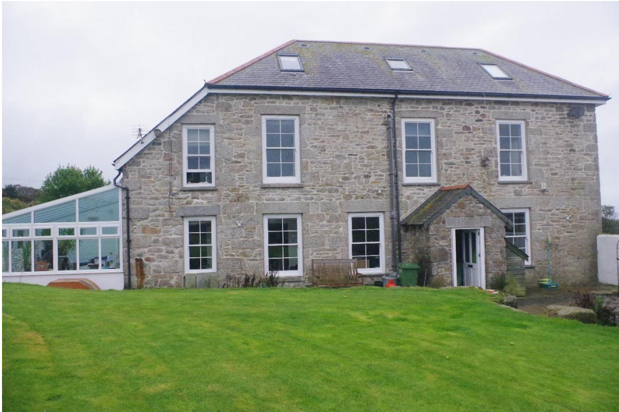
Fig 9 View of the east elevation of The Count House from the garden.
