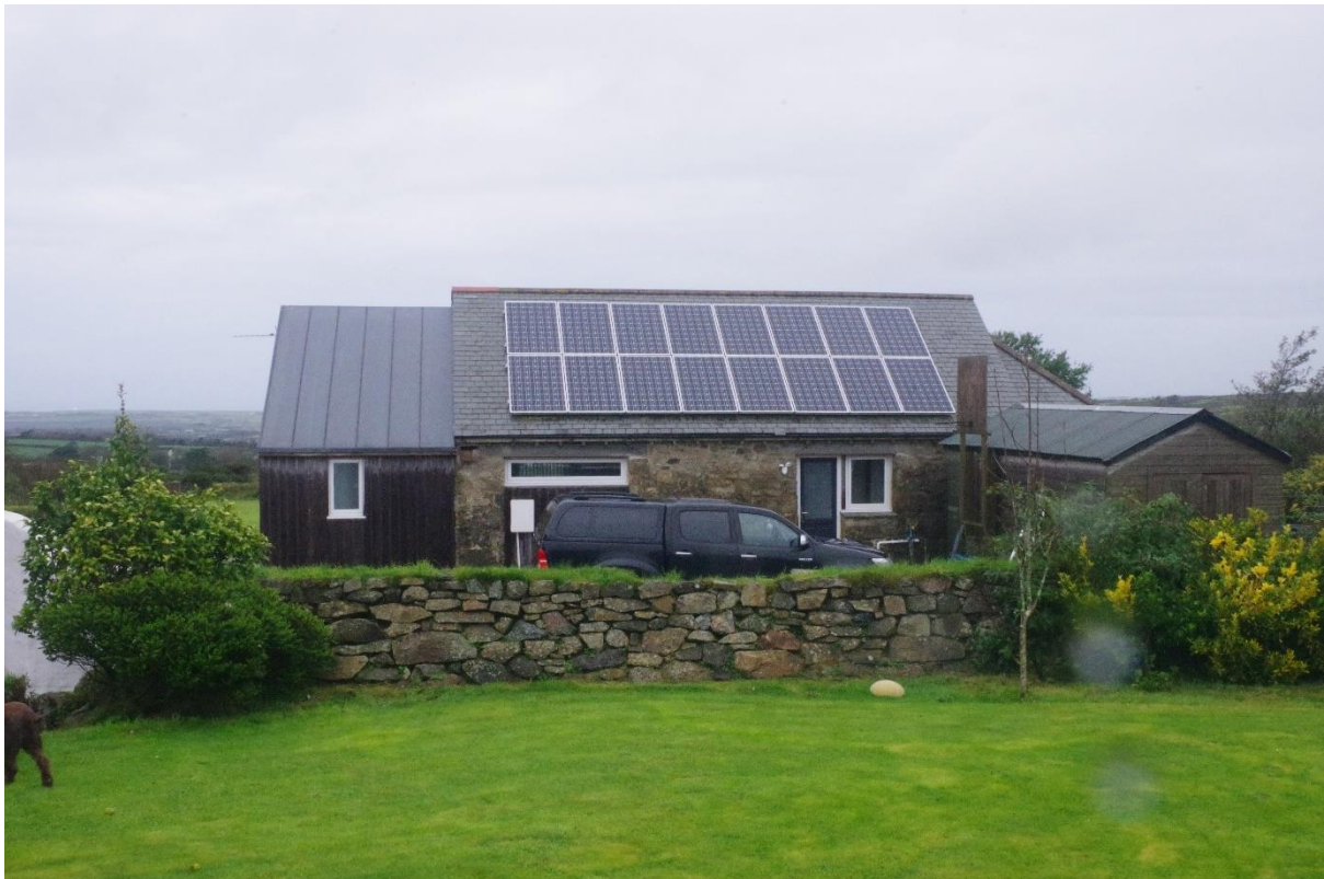
Fig 16 View from the garden in front of the east elevation looking north to the converted late 19th or early 20th century outbuilding.
