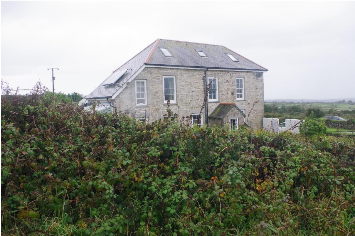
Fig 11 View of the Count House looking north-west from the footpath.
