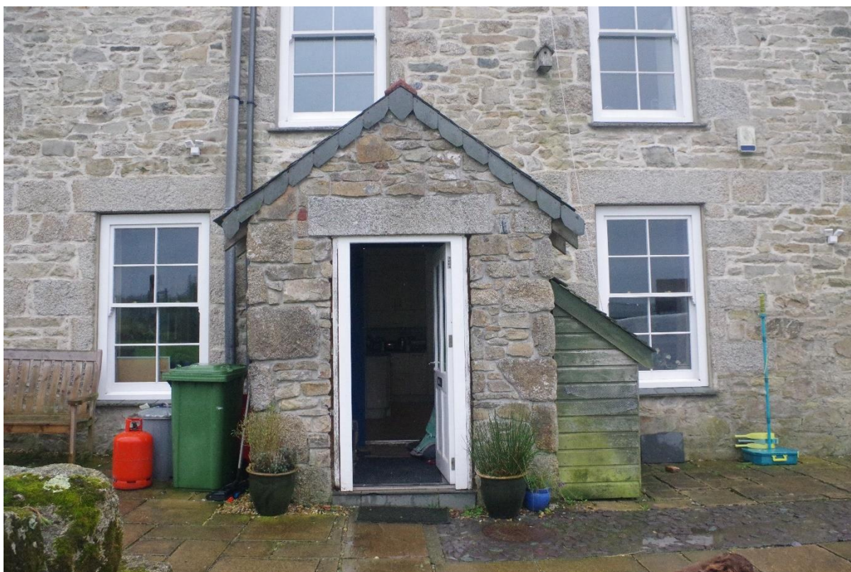
Fig 13 Existing modern stone-built porch.
