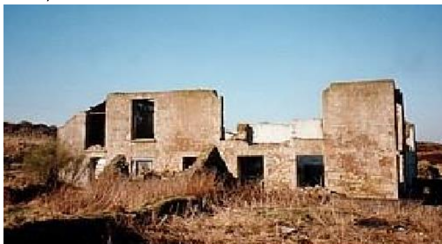
Fig 8 East elevation prior to rebuilding in 2000.
