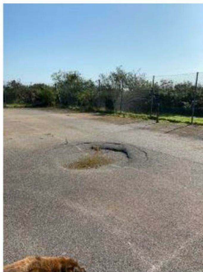
PHOTOGRAPH 2: View of a mine shaft within the central area of the site
