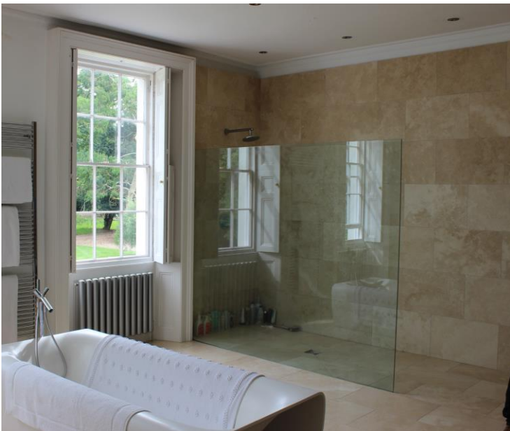
Existing ensuite, travertine tile walls & floor, modern cornice
