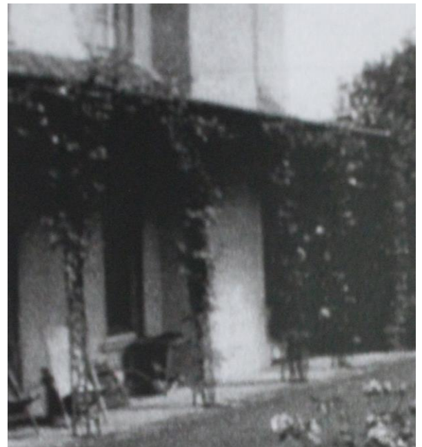
Historic photograph of the south elevation of Wyddial hall showing metal framed veranda.
