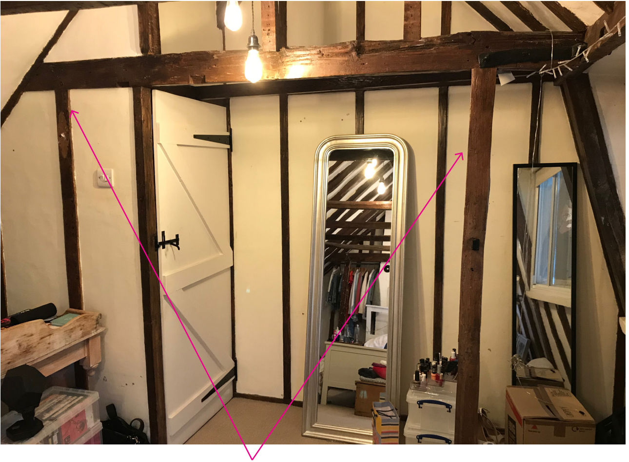
Existing arrangement showing original vertical posts, which will be kept in place
