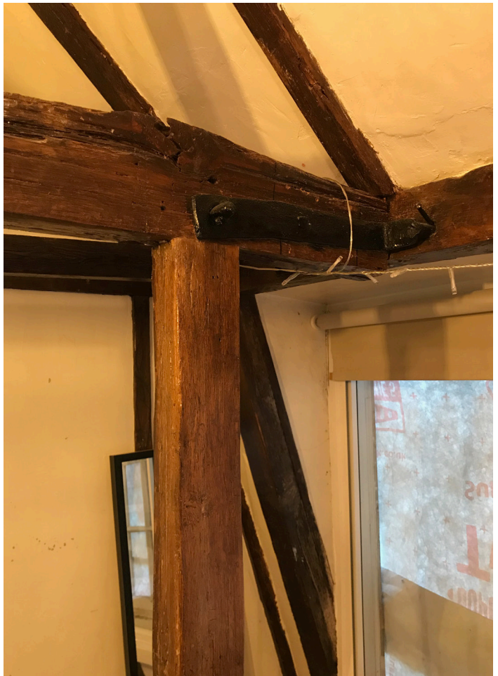
Existing arrangement showing original vertical posts, which will be kept in place
