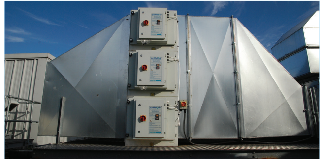
3 ESP Units Stacked in modular formation
