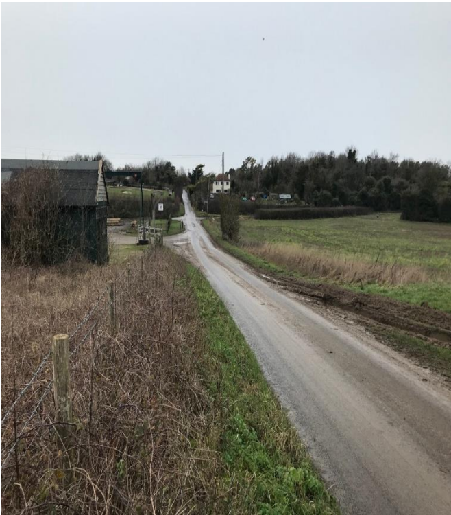
Exit view looking towards Shepherdswell
