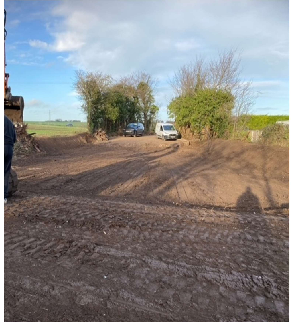
Figure 7 Photograph of the site currently
