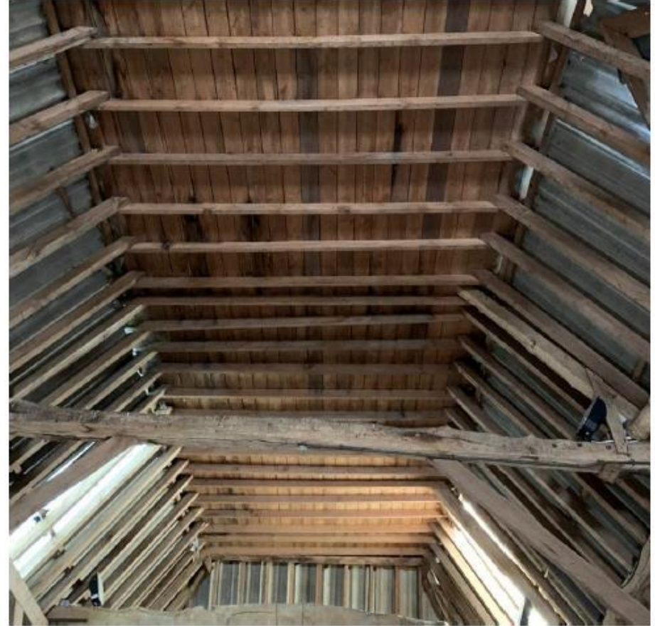
Photo of the 1960's roof which has replaced the original roof.
