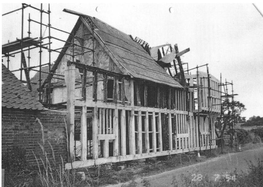
1990s restoration works - Beech Architects (2016)
