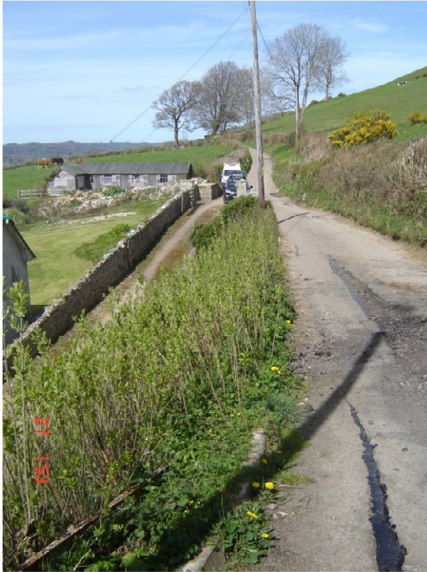
View along Nower Road at top of retaining wall.
