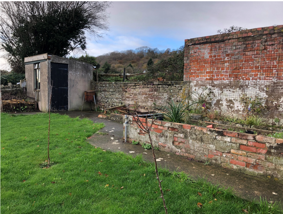
Dilapidated structure at the rear of the garden
