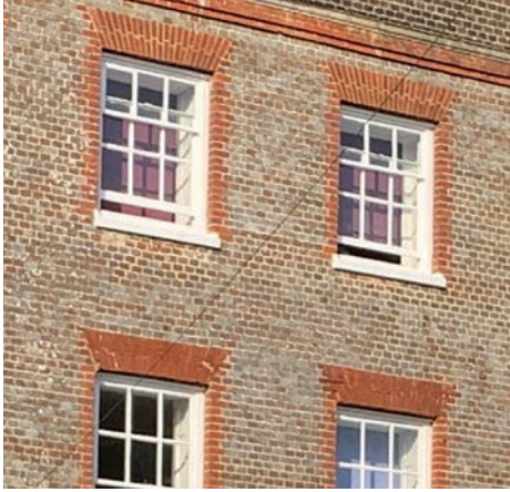
Brick and Flint represents a significant portion of the village with Georgian windows
