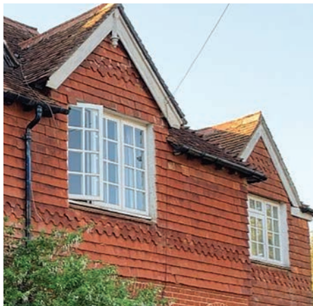
Tile Hanging again gives a traditional feel to the building. These could be reclaimed tiles to add age?
