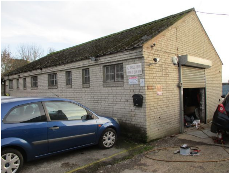
Photograph 1: Building B1 as viewed from the northwest.
