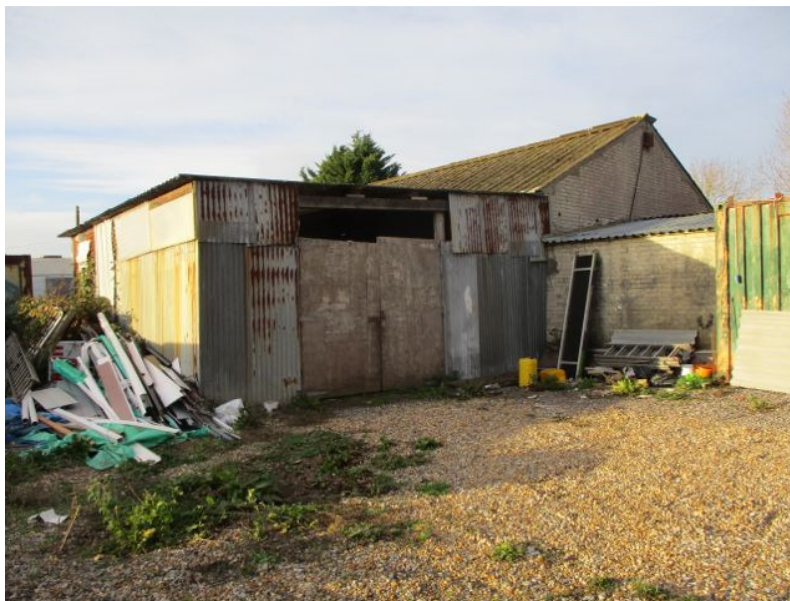
Photograph 2: Building B1 as viewed from the southeast.
