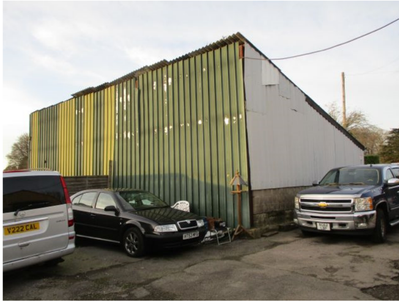
Photograph 5: Building B2 as viewed from the southeast
