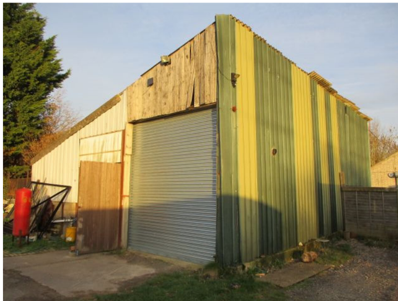
Photograph 6: Building B2 as viewed from the southwest.
