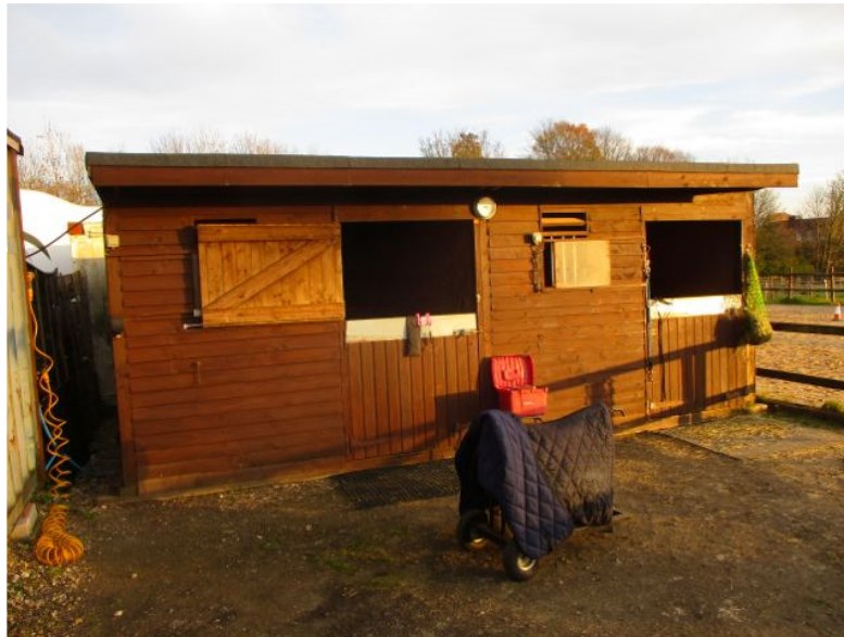
Photograph 8: Building B4 as viewed from the northwest.
