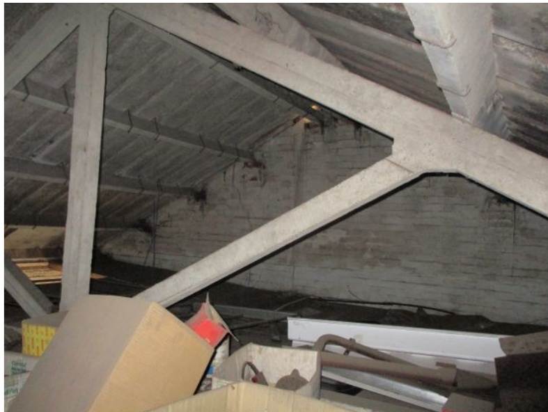
Photograph 4: Typical views of the interior of B1 (roof space).
