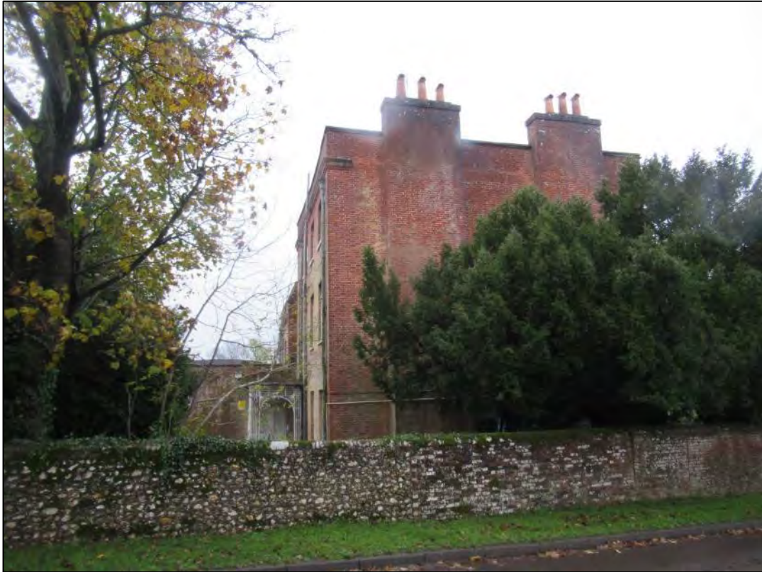
Plate 13: View of western elevation of Catherington House
