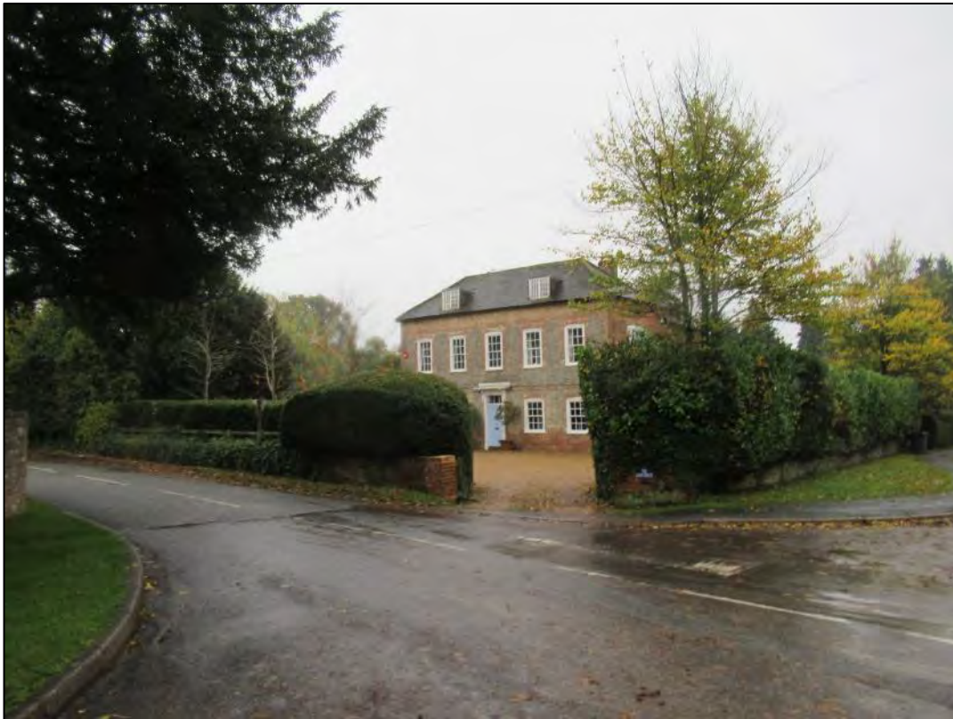
Plate 15: View towards The Farmhouse from the north west
