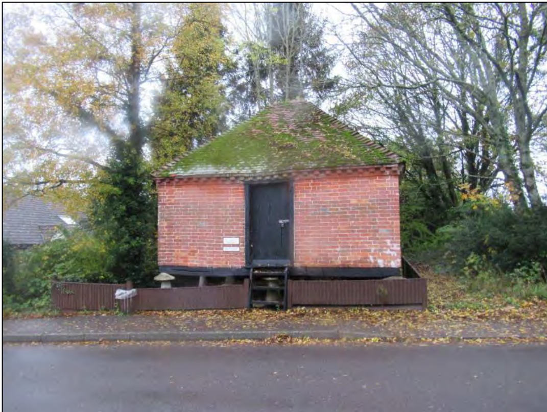
Plate 16: View towards the granary
