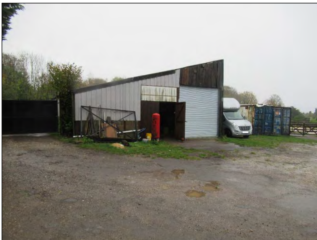
Plate 4: View across the Site towards the east
