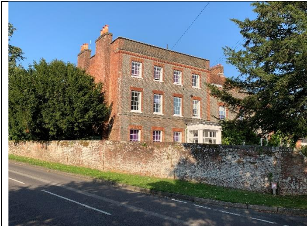
Kings Court School, a grade 2 Listed Georgian building (formerly Catherington House) is to the South East of the site.
