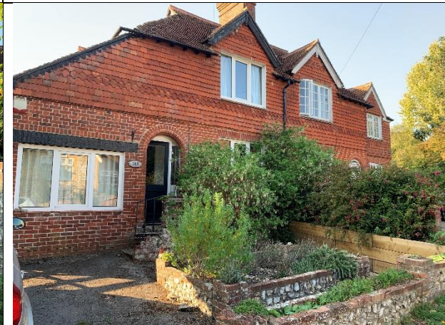
Red brick and dark tiled roof is a common feature as is tile hanging.
