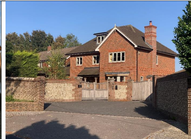
New property to the North East of the site built in traditional brick.
