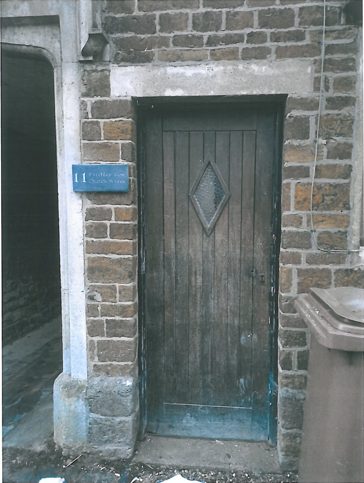
EXISTING FRONT DOOR
