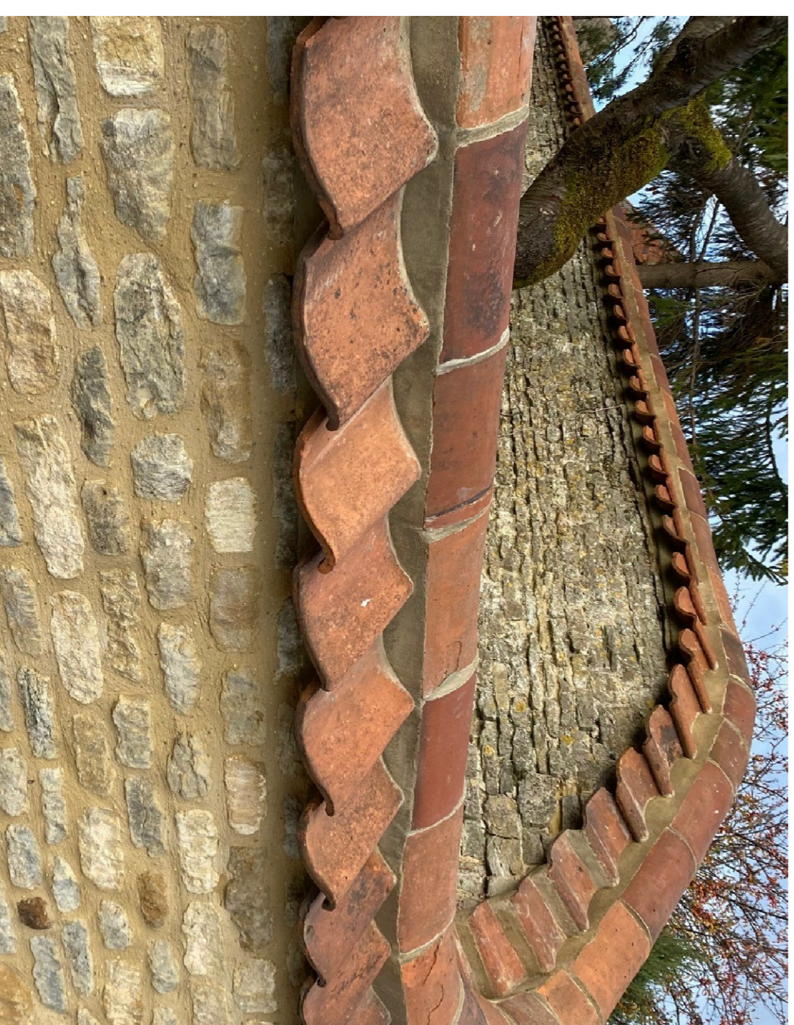
Photo showing proposed finish to Annex coping
