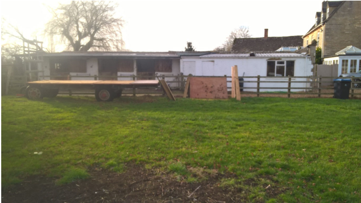
North-east elevation of former garage and stables outbuilding to east side and rear of main house, now demolished.
