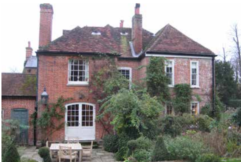
The house viewed from the west; parts of the the range to the right perhaps date from the 16th or 17th century
