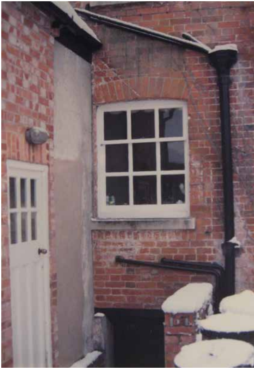
The larger projection, c.1986; note the external basement steps (centre bottom), and the 'scar' showing the pitch of the glazed roof that once provided shelter to the basement steps
