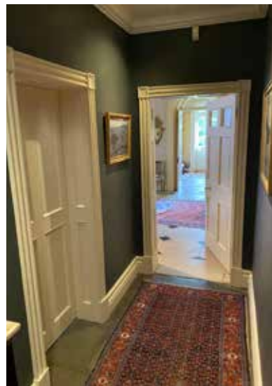
View east along the corridor; the door to the left is that to the present cloakroom; all the joinery and cornicing is modern
