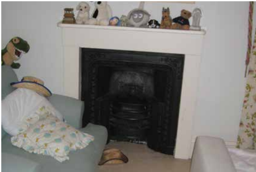
The early 19th century chimneypiece in the first-floor bedroom to the west of the principal stair compartment
