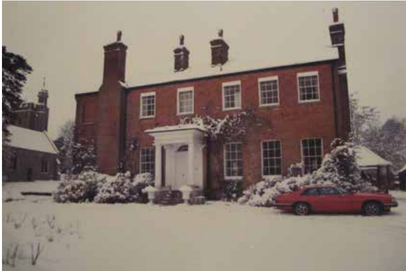
The eastern elevation, c.1986; note the two blind windows to the left of the face-fixed chimneystack
