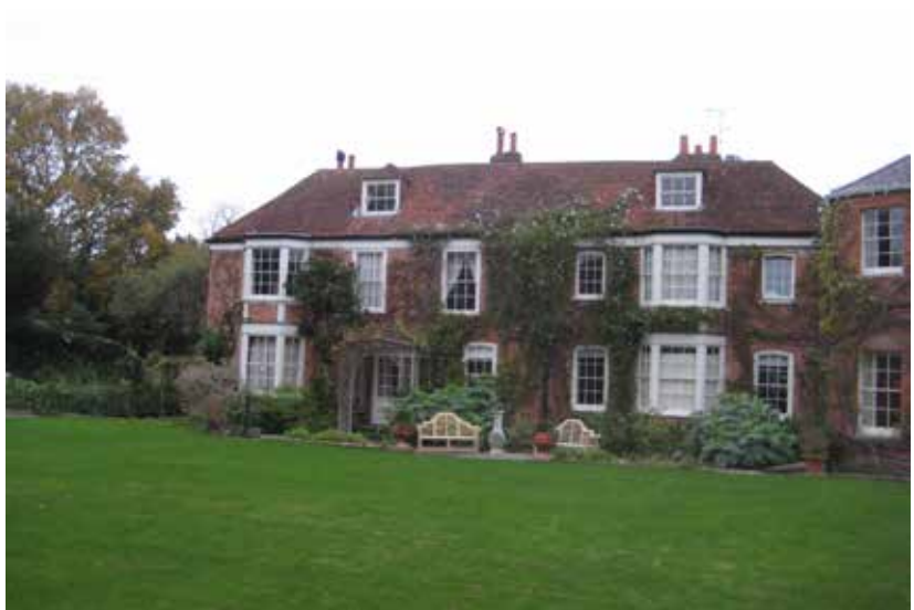
The volume containing rooms A, B and C, left to right, viewed from the south
