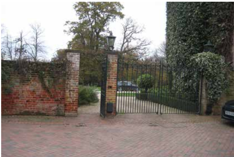
That part of the north-south wall adjacent to the house, including the three gatepiers, was entirely reconstructed in the late 20th century
