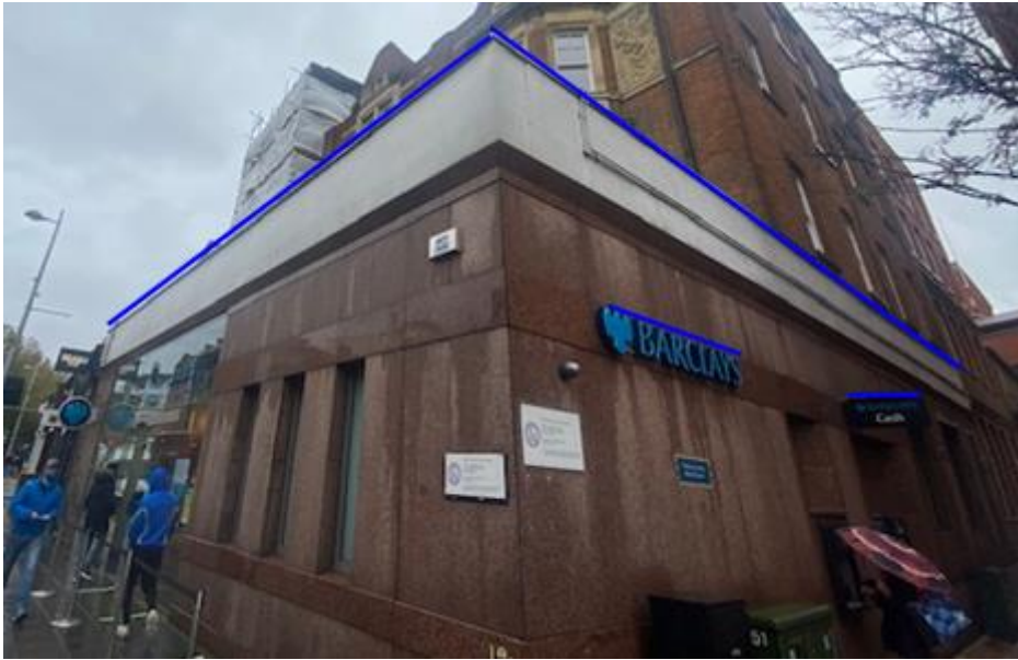
Image 4: Blue line shows the proposed location of the bird deterrent spikes to the eaves and on the advertisement signs.
