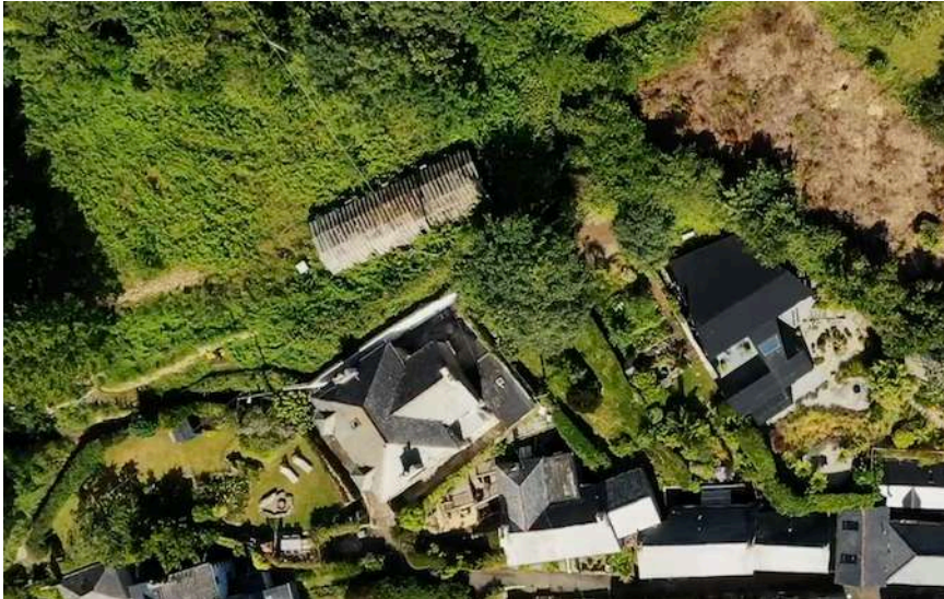
7 EXISTING BUILDING AERIAL IMAGE - 14.6M LONG X 5.8M WIDE
