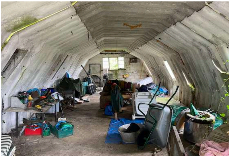
6. EXISTING BUILDING INTERNAL - 14.6M LONG X 5.8M WIDE
