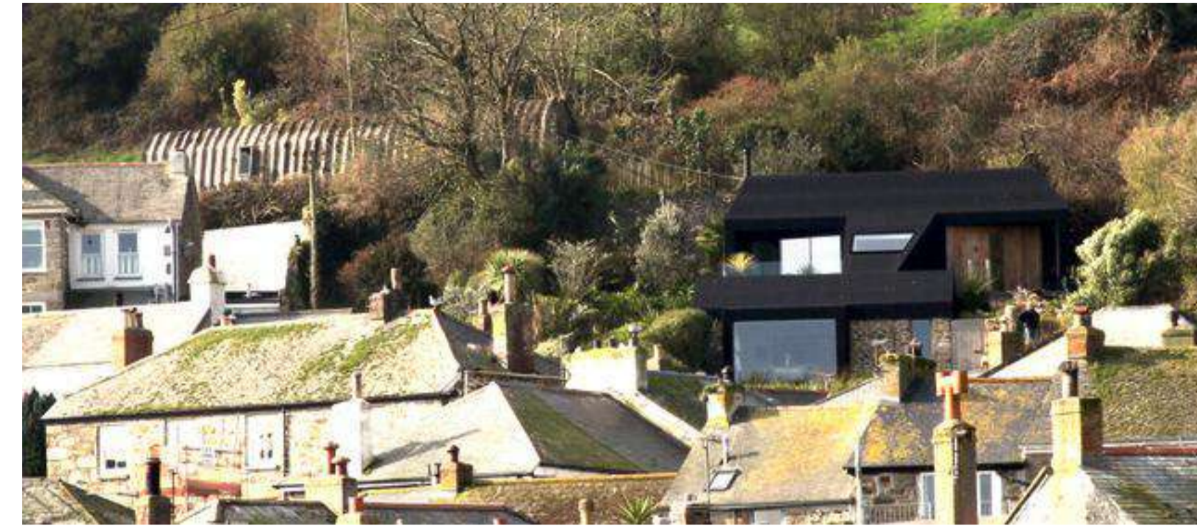
Photo from East - As Existing
