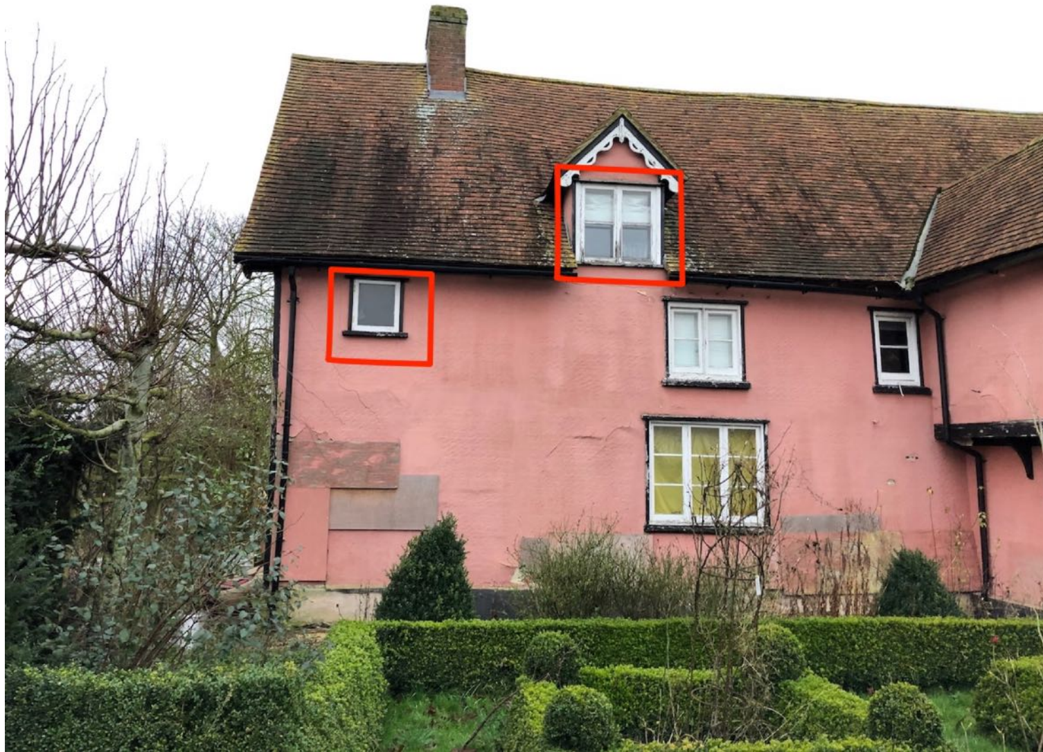
West elevation showing 2 no. windows to be replaced
