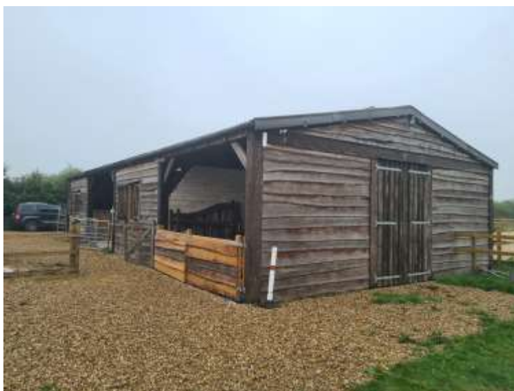
Figure 1: General View of the Stable Building
