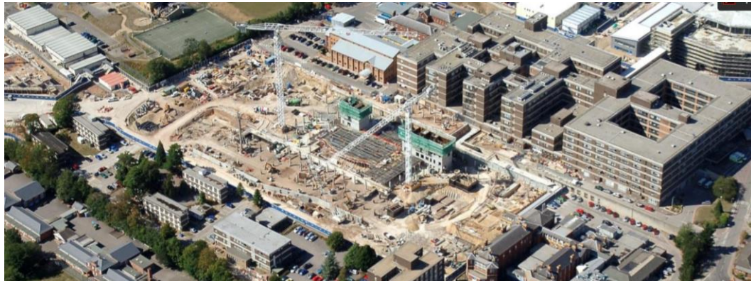
AUGUST 2006 AERIAL VIEW
