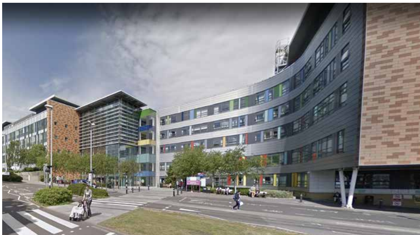
Queen Alexandra Hospital main building
