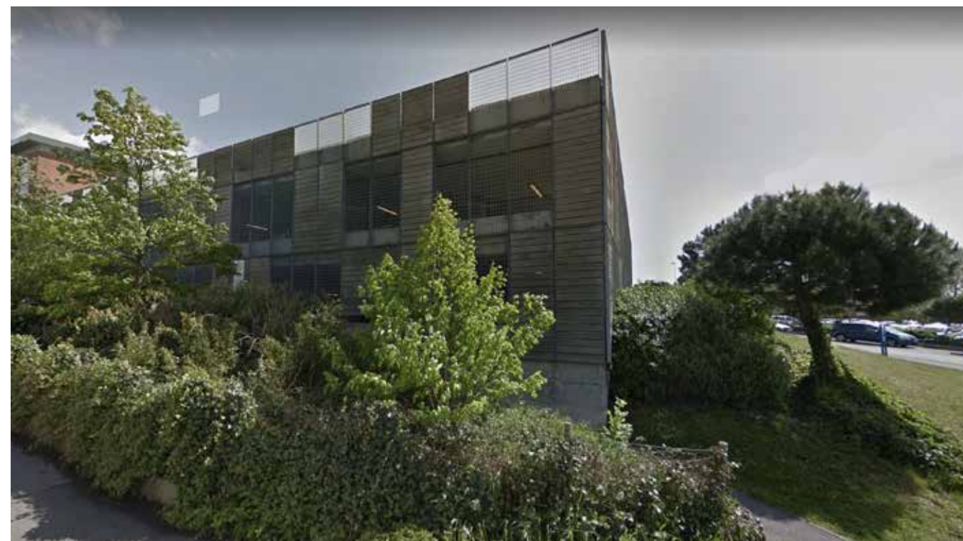
Main entrance car park
