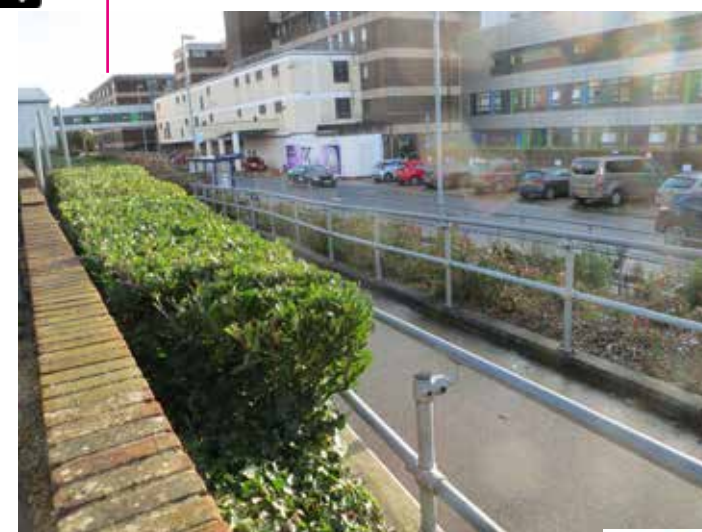
Existing pedestrian ramp
