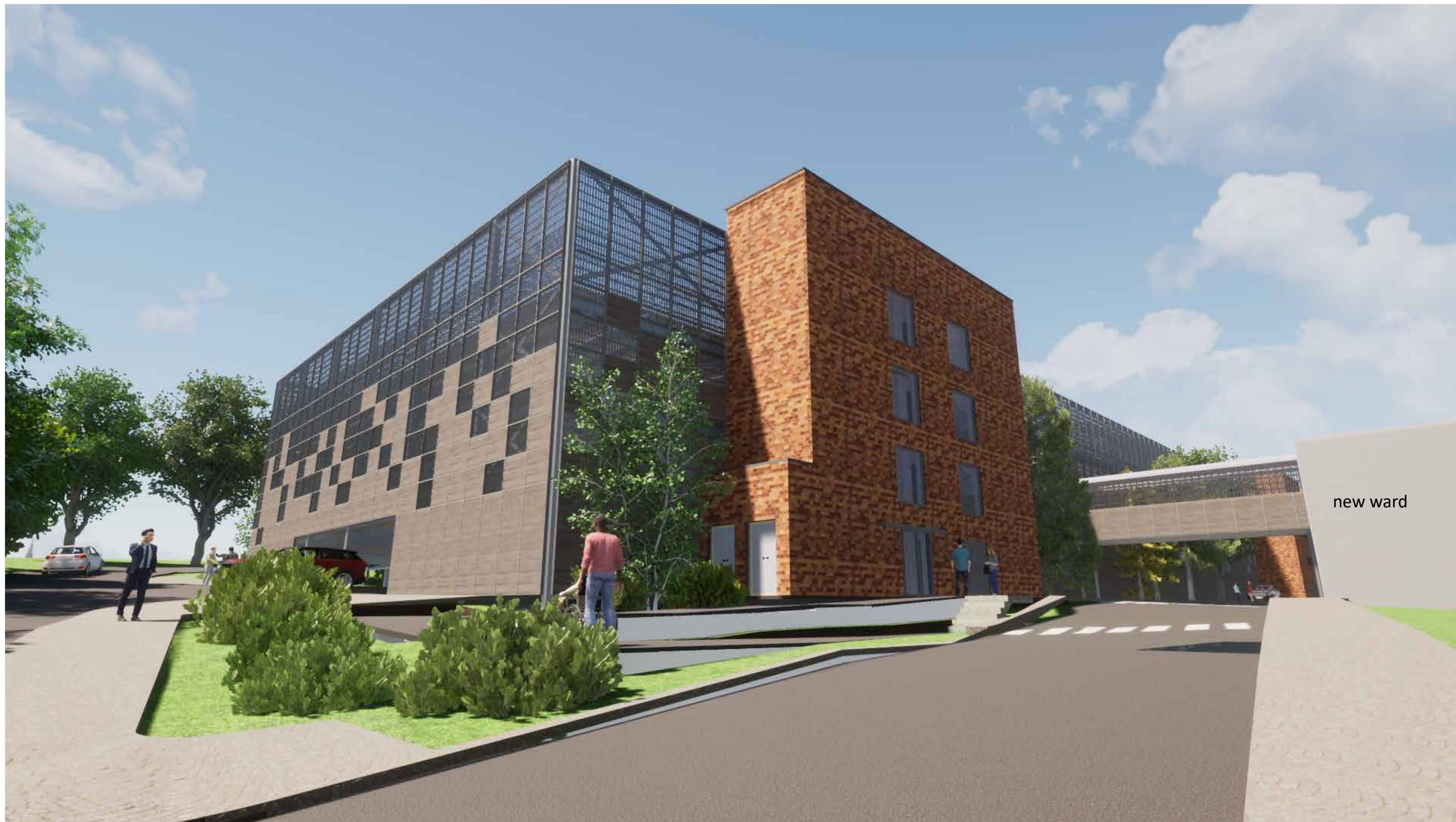
Computer Generated Image from Harvey Road, looking at the south and west elevations.
