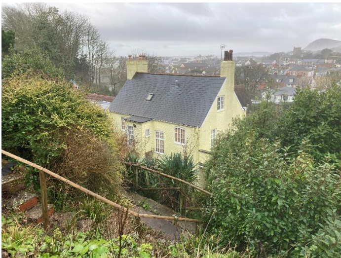
Figure 2 View of the rear of the property from Beatlands Road
