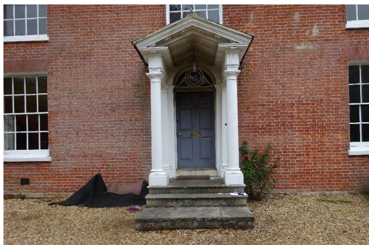
Elevation to front porch.
