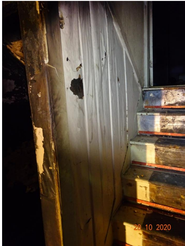
Cladding of the wall between the stairs to bedroom 5
