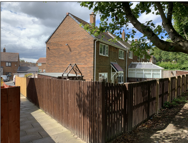
Photo 3 : Rear of property viewing southwards down footpath
