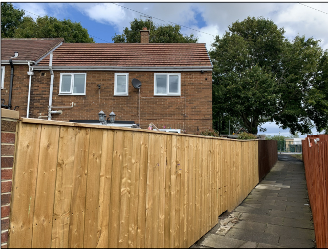
Photo 1: Front of property viewing northwards down footpath
