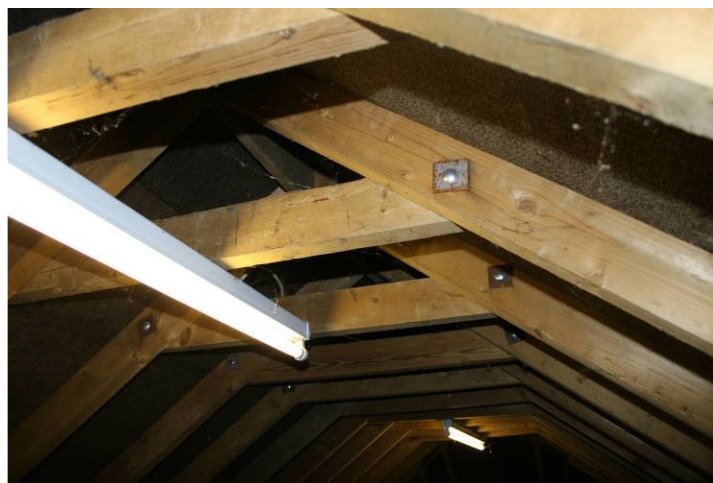
Photo 11: Large storage area above garage
