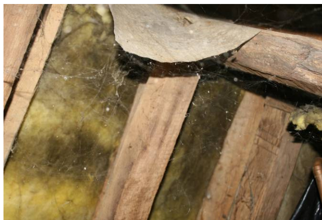
Photo 3: Shallow ridge void with water tank. Fibre glass under-felt
