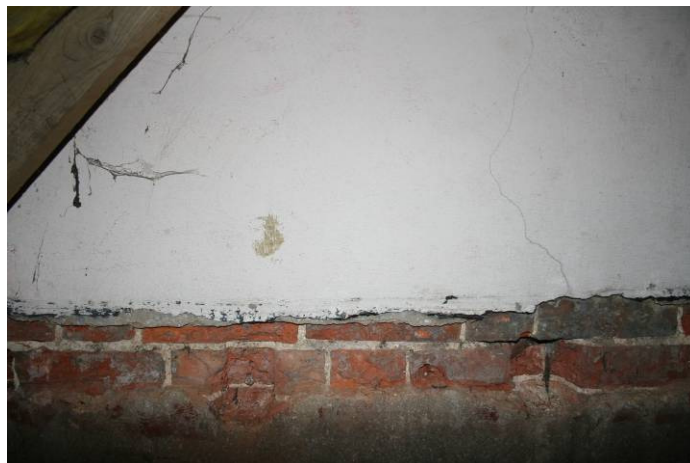
Photo 7: Former external wall of cottage within roof space of extension
