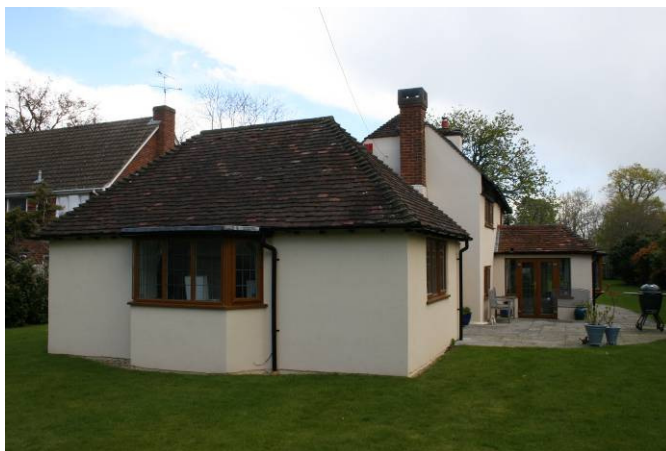
Photo 4: Western extension linked to the main cottage in the 1970's
