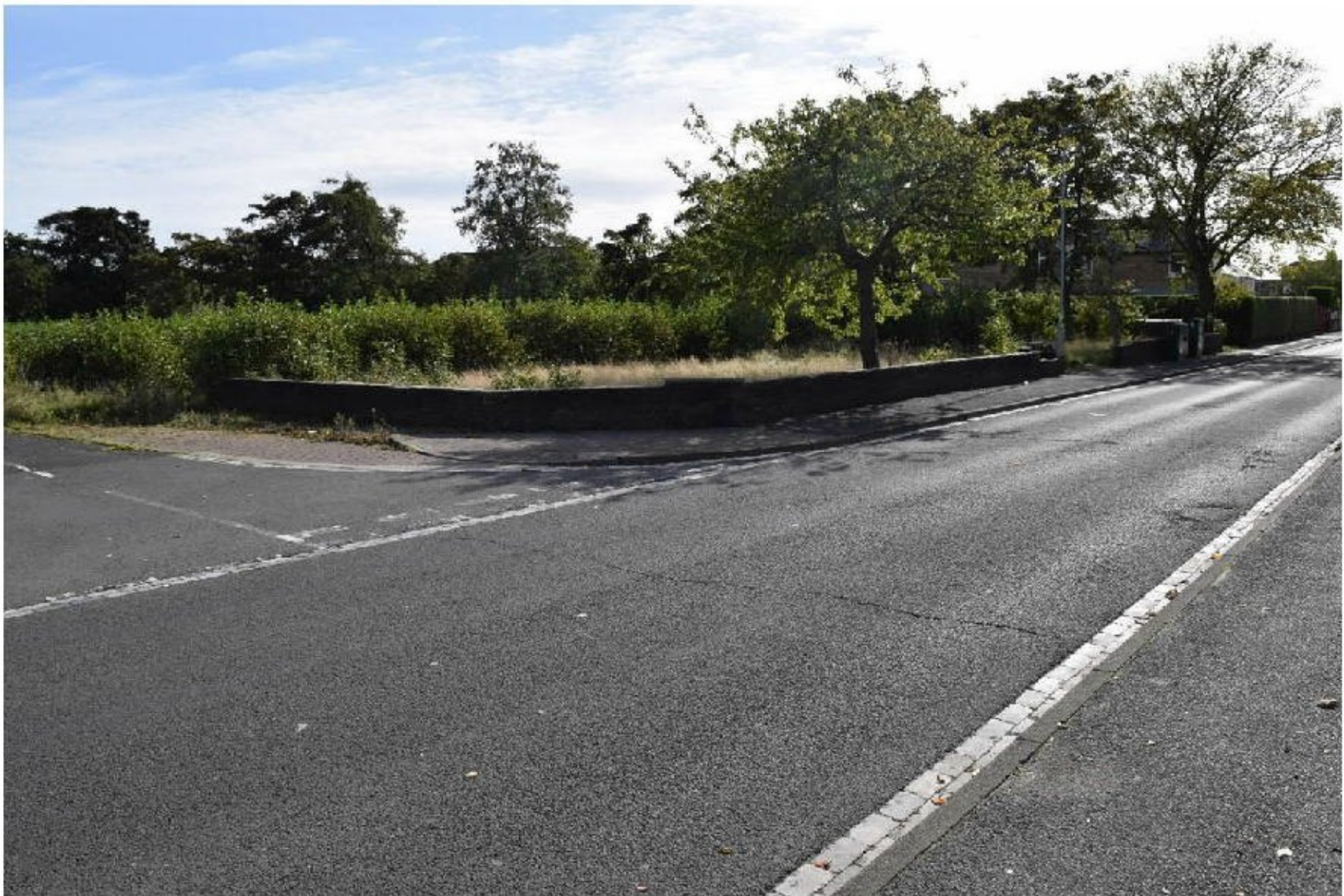
Plate 8. View of the boundary wall and access at the west side of the former site of Essendene Care Home within the Site, looking south-east.
