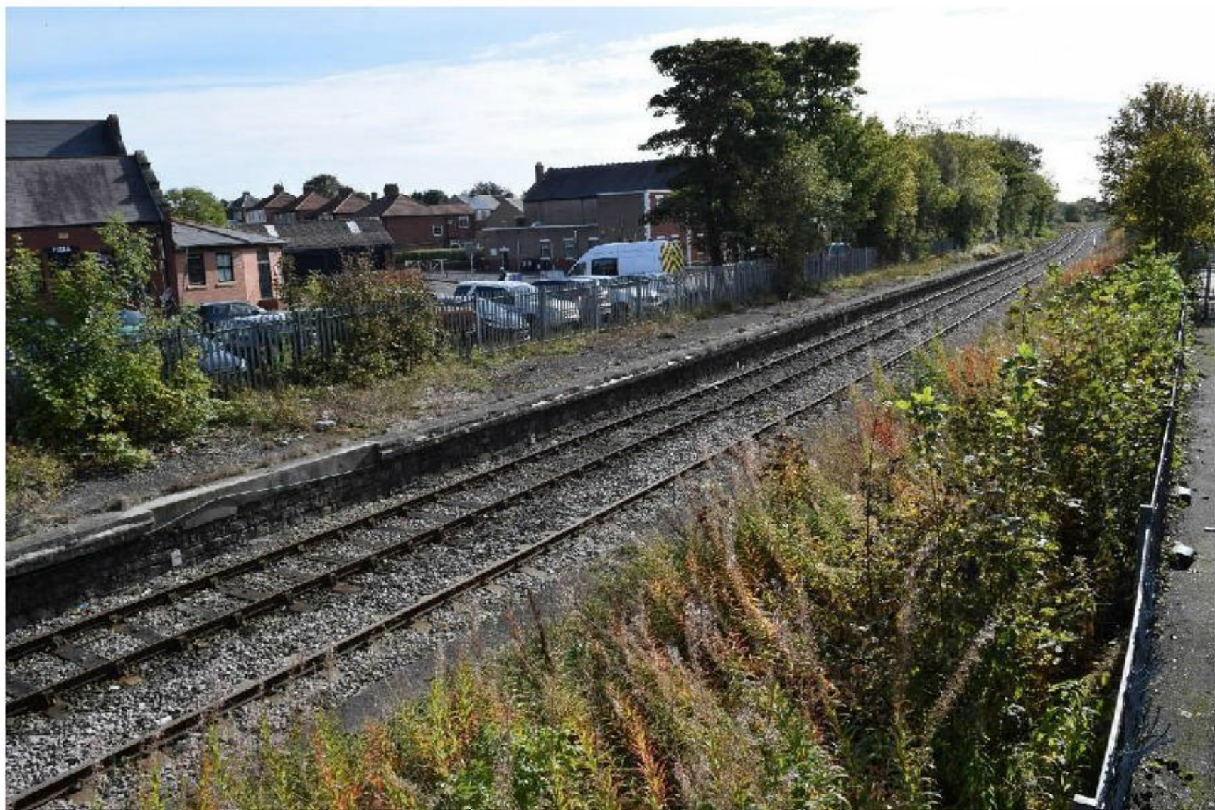
Plate 10. View from the access ramp over the existing railway line and redundant stone platforms of the former Ashington Station [HNER 27333].
