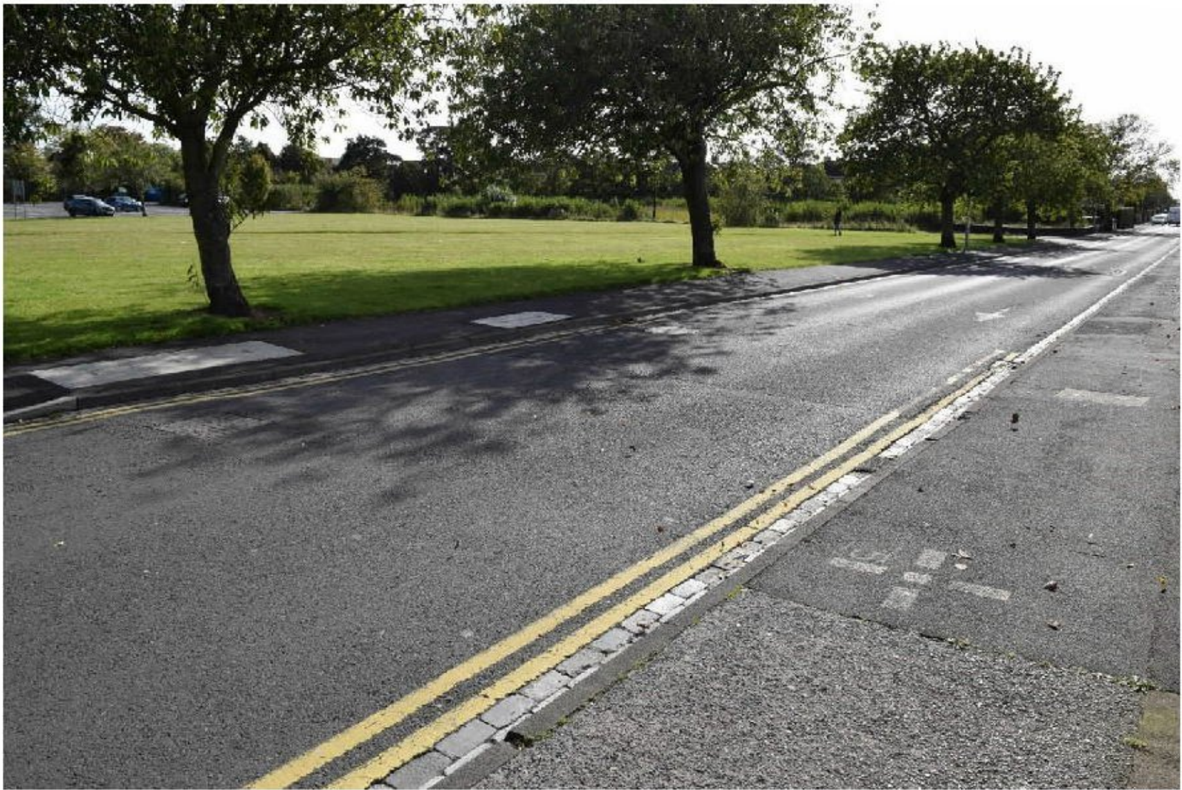
Plate 7. Detail of services in Kenilworth Road to the west of Library Gardens and associated slightly raised area within the Site, looking south-east.
