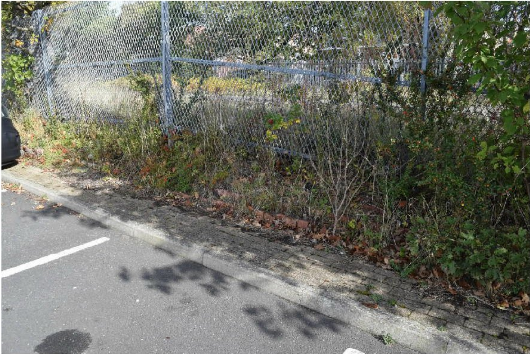
Plate 5. Detail on the basal courses of a building [AEC010] on the east side of the Station Yard South carpark within the Site, looking north-east.
