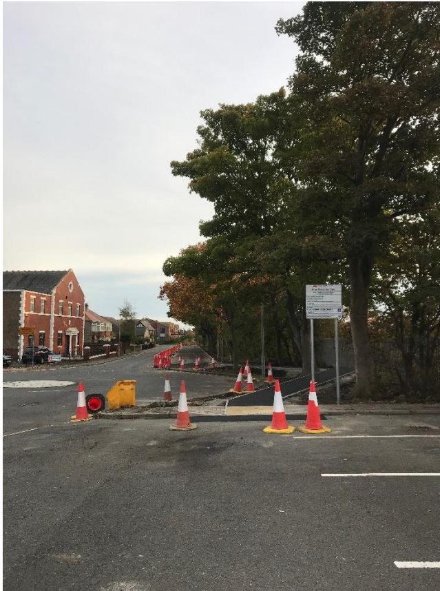
Figure 6. View south down John Street.
