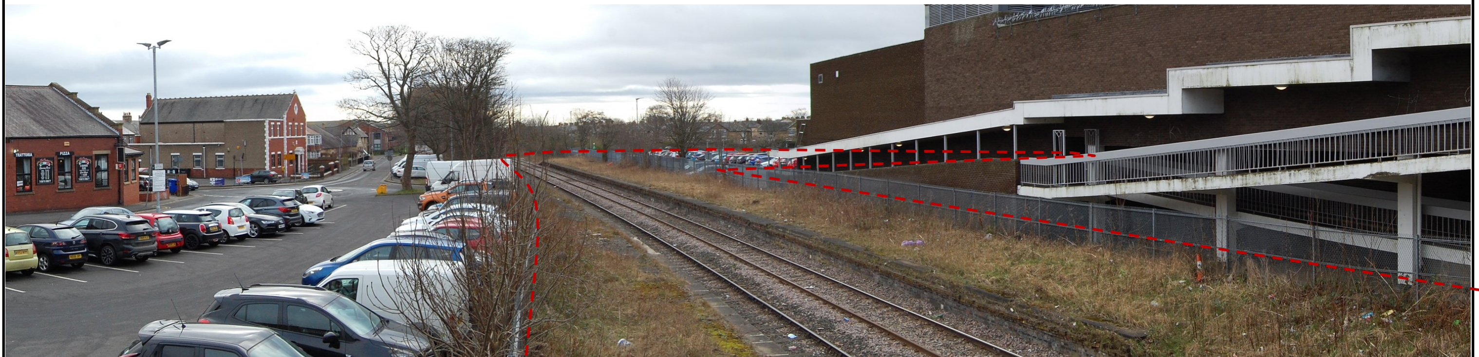
View 5: View south from steps of pedestrian bridge
