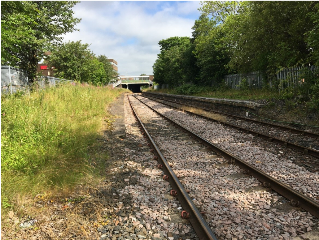
Plate 1. Northumberland Line looking north west from southern portion of the site area.
