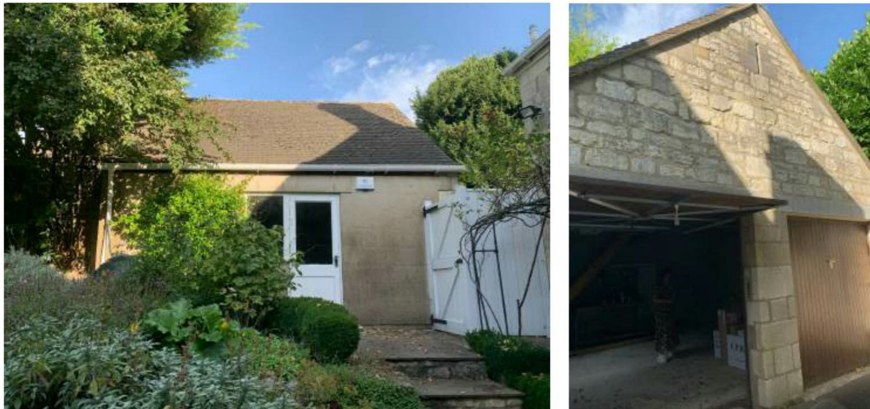
Photographs of the existing garage building.
