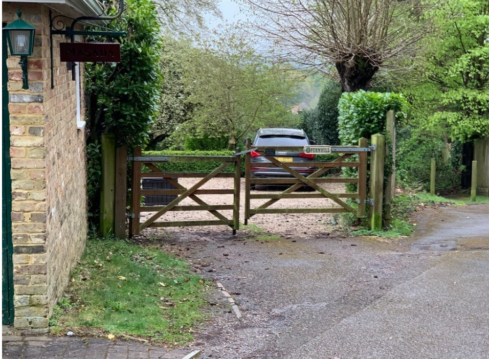
Fig. 1. Existing Entrance Gates
