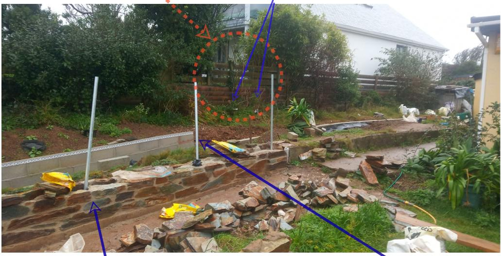
500mm-high stone wall (under-construction) with vertical holes concreted in for galvanised fence supports (here, for illustration, just resting in place before permanent fixing). Fence to be 1.20m high, as per D&A statement. (The 1.2m fence tops the low wall which itself replicates the level change between lawns visible in photo 1 of DAS.) Fence to extend to right in this photograph, to garage.
