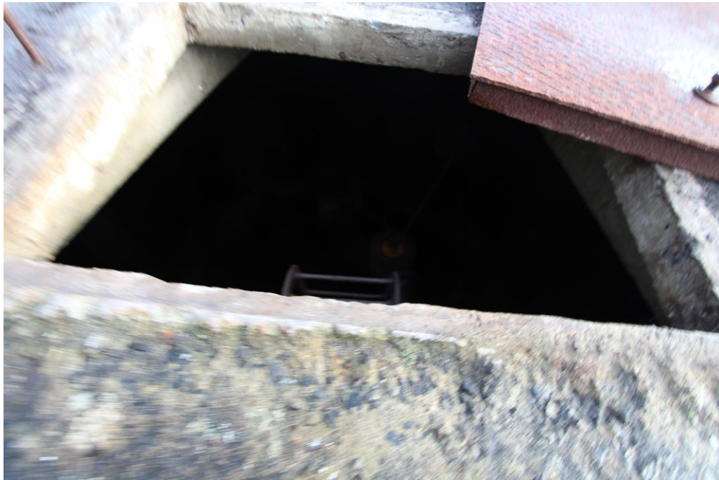
Access hatch in roof.
