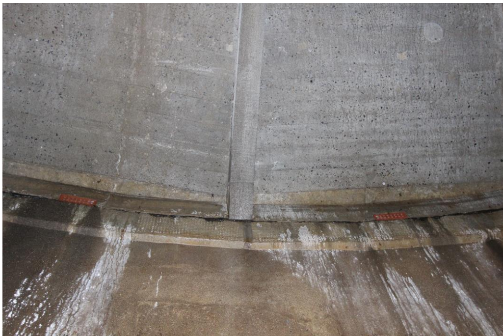
View up wall to junction with roof and ring beam
