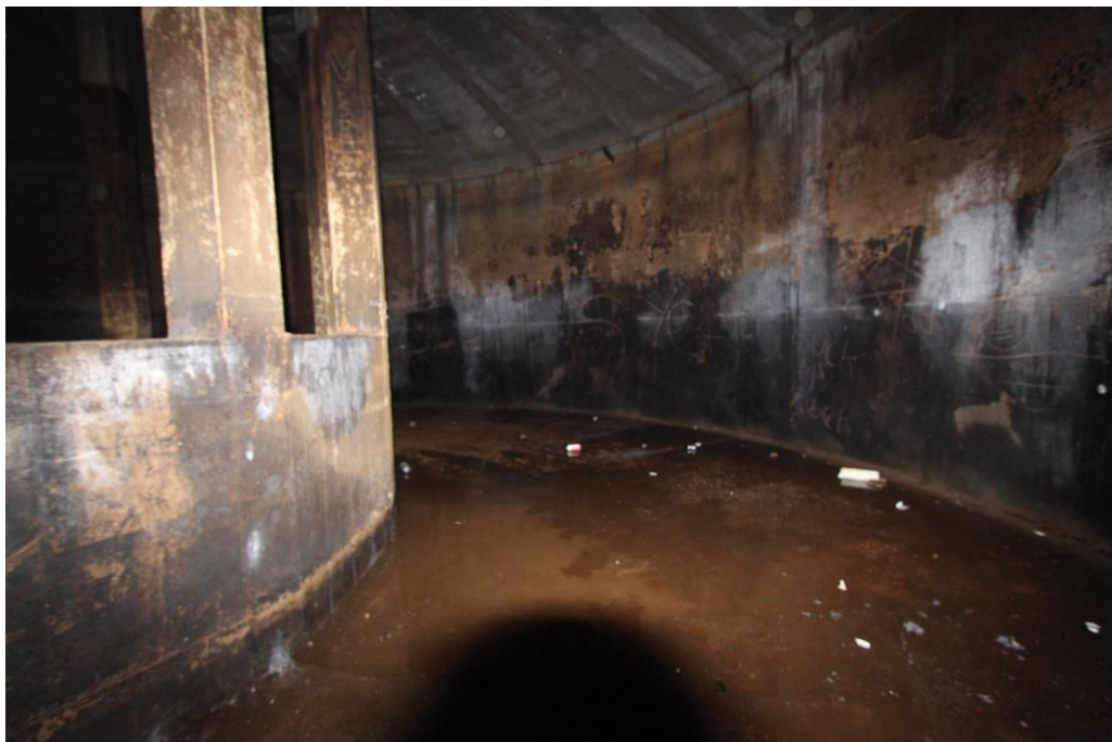
View of central columns and external wall. Wall staining is not rust from the reinforcement.
