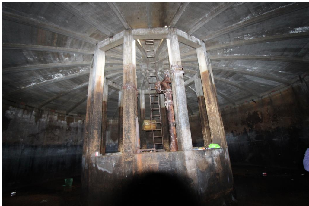
Central ring of columns supporting ribs in roof.
