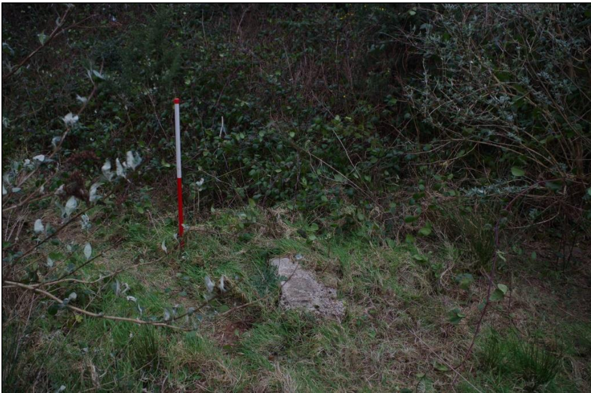
FIGURE 12: POSSIBLE TRACE OF BOUNDARY WALL TO NORTH OF THE WATER TANK; VIEWED FROM THE SOUTH (1M SCALE).
