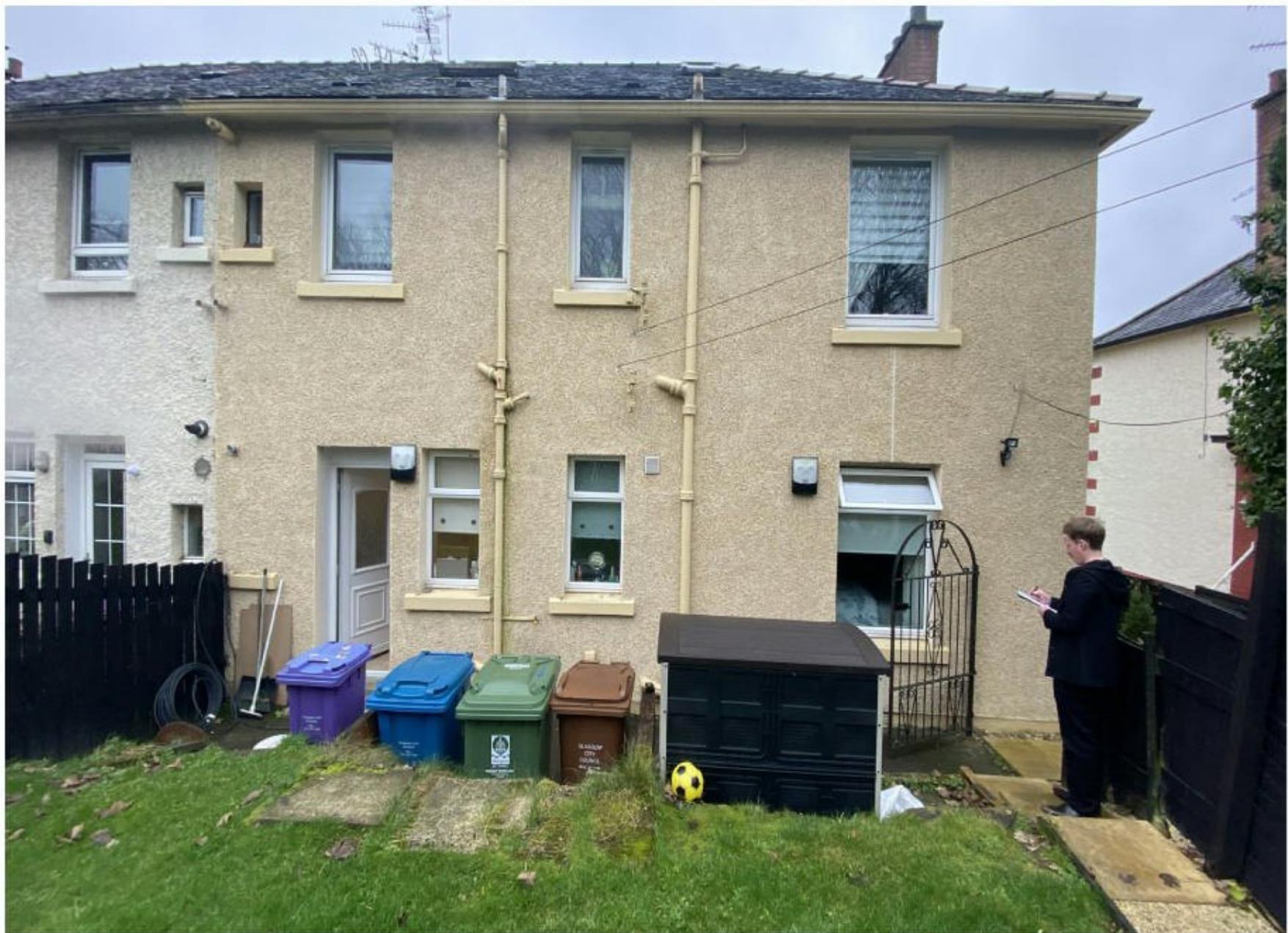
28 BRORA STREET REAR FACADE
