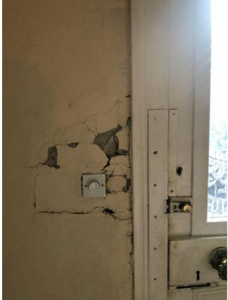
Stone is saturated through to the inside of the building. Shown here is the inside of the building, next to electrical switch. The plaster has lost its key and is crumbling away from the wall
