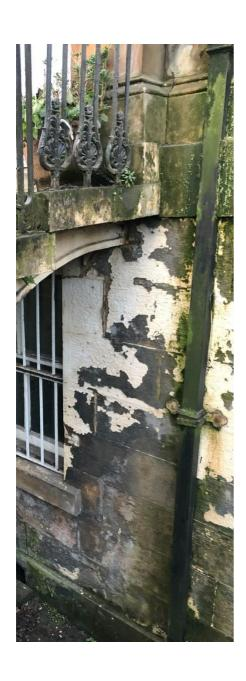
Hopper also needs to be replaced, slightly increased in size to be able to cope with increased rainfall.
