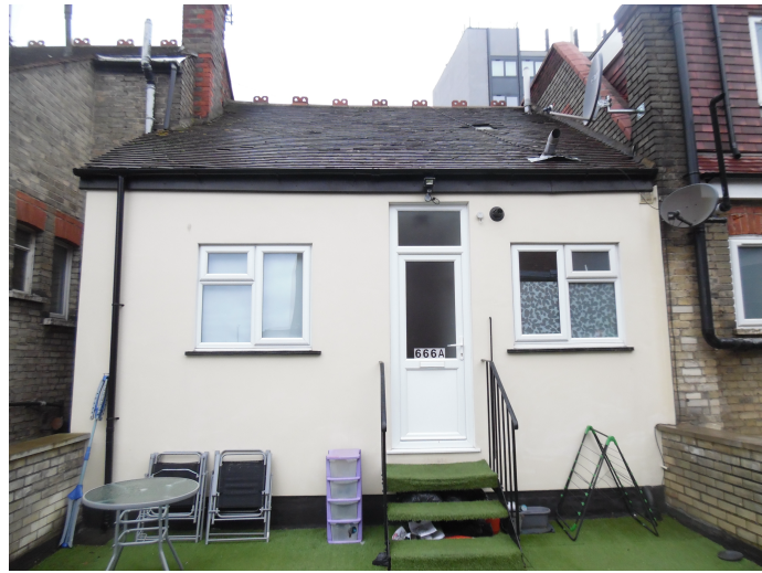
Rear view from ground floor's extension roof
